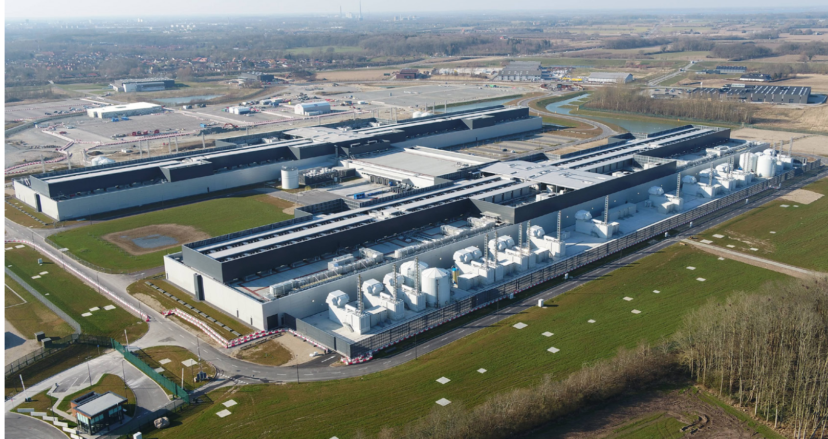
Facebook Odense Data Centre, Odense, Denmark
